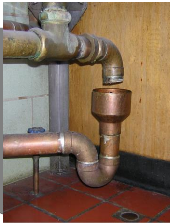
Side view of an indirect connection using a funnel drain
